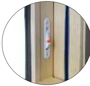
Window Operating Control Device
